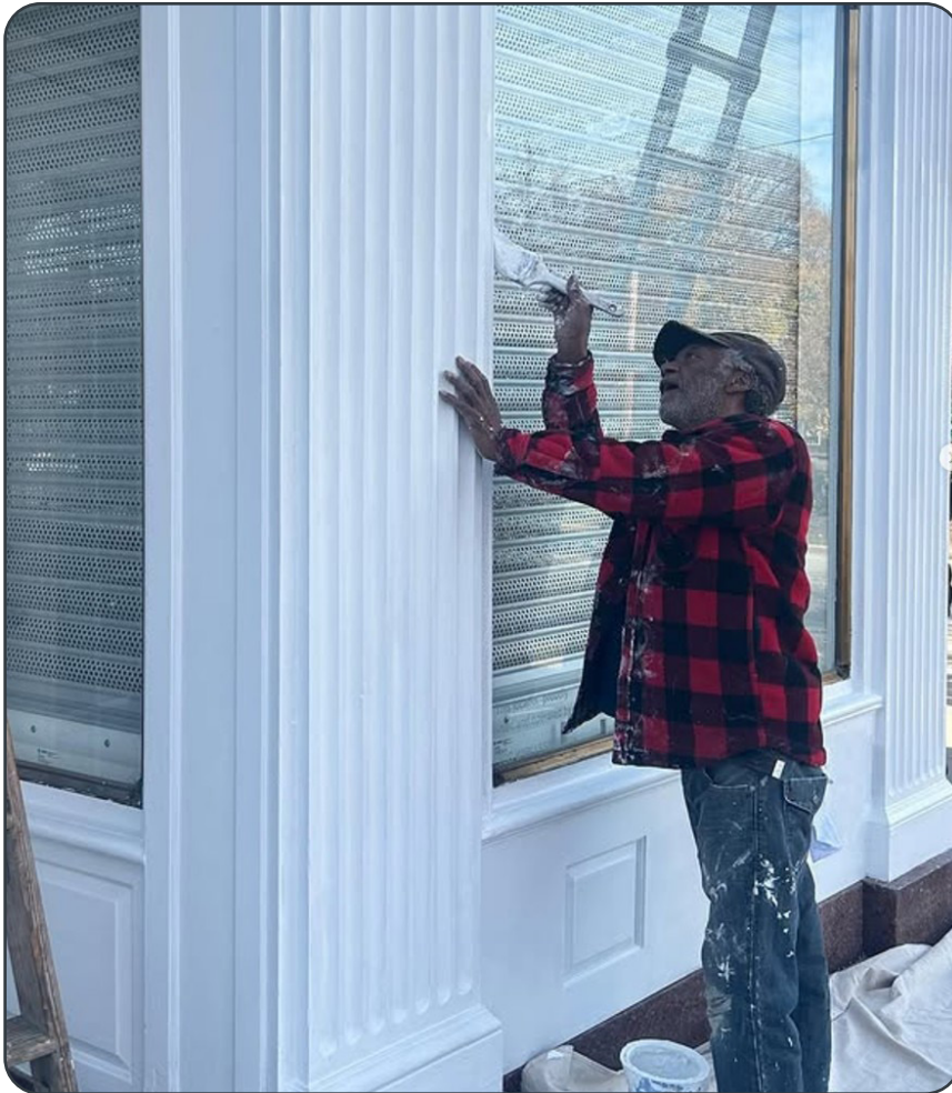
$5 million in basic maintenance upgrades, from roofs to HVAC
